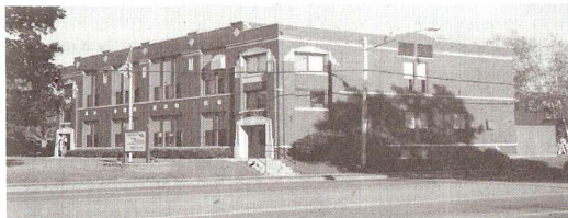
1. Community Center (Langlade County Teachers Training School) - 411 Superior Street (1925/26) at a cost of $53,440, teachers trained there through 1971. Built of Bedford stone, it included a gymnasium with a spectator balcony, an auditorium, and classrooms. It now houses the Langlade County Department on Aging.
