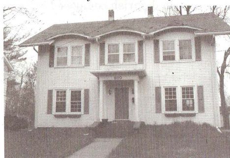
5. Sears Roebuck Kit House - 810 Seventh Avenue - This is one of several "kit" homes in the area. In the late 1800s and early 1900s, several companies made these kits for all types of buildings. They would ship components by rail in the order of use for construction. Prices varied with the extras ordered, but the average basic price was $3,278.
