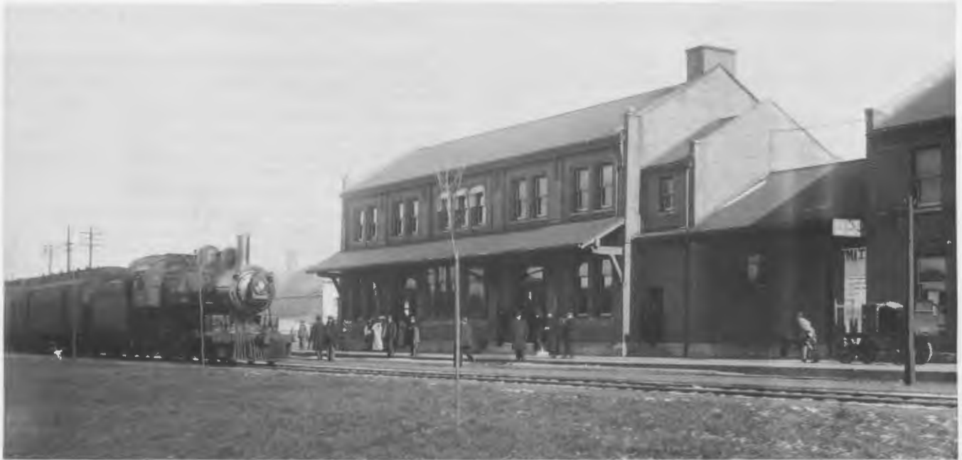
High noon at Antigo in October, 1907. The new depot has just been completed and the Ashland Division offices now occupy the second floor. Train 116, pulled by engine 200, a class B, 4-4-0 type, is arriving from Ashland and will stop for fifty-five minutes to enable its passengers to have lunch. The "lunch" sign is evident on the corner of the building on the right side of this photo. The covered space between the two parts of the depot was eventually walled in. Photo from the collection of Russ Porter.
