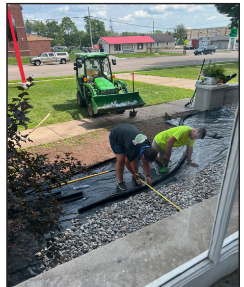
Fischer Maintenance installing mulch on the museum grounds main facade
