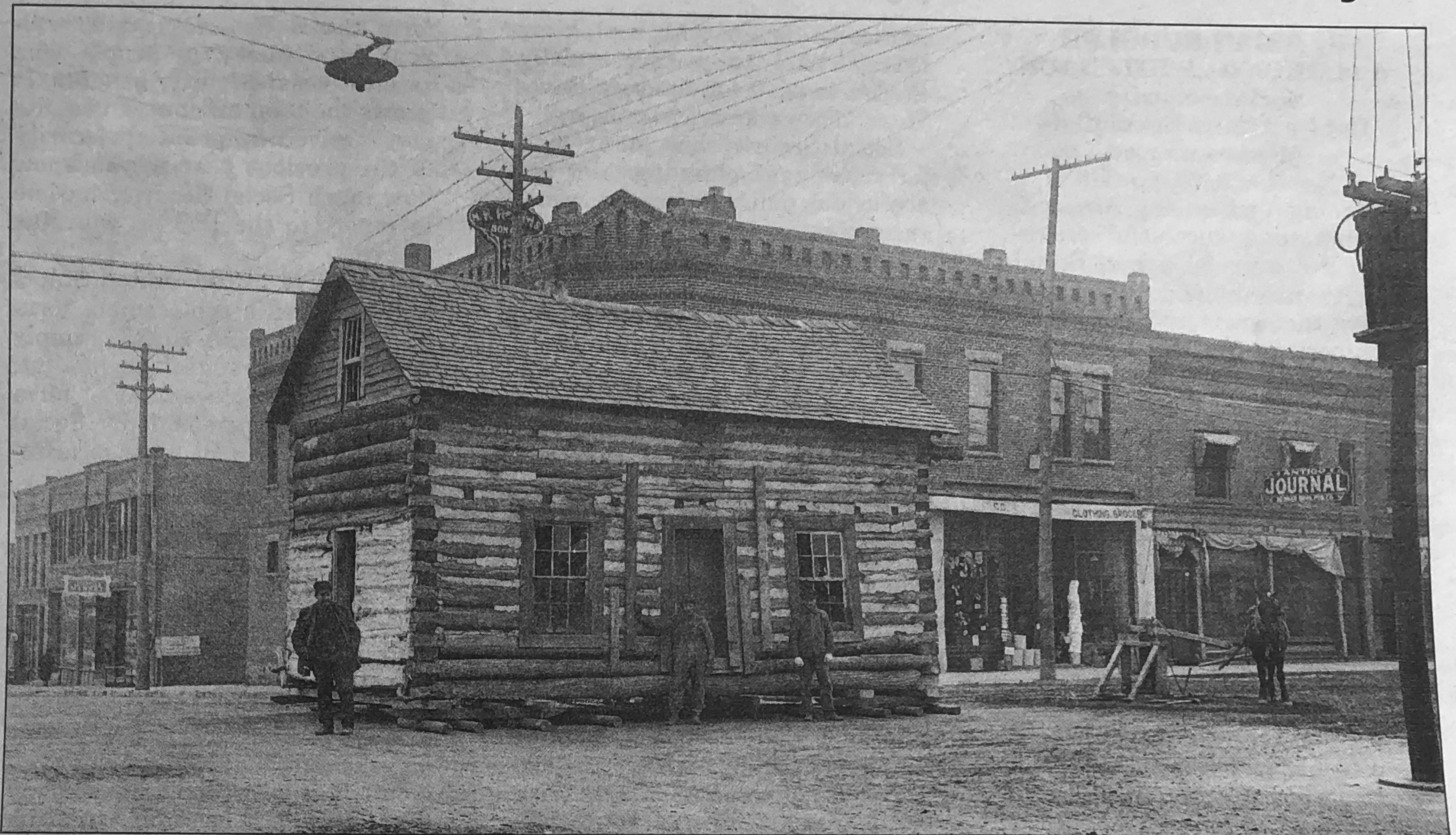
In 1914 Antigo's first home, the Deleglise cabin, stood in the way of downtown development. Rather than tear it down the city put it on log rollers and wheeled it down the road to the library.
