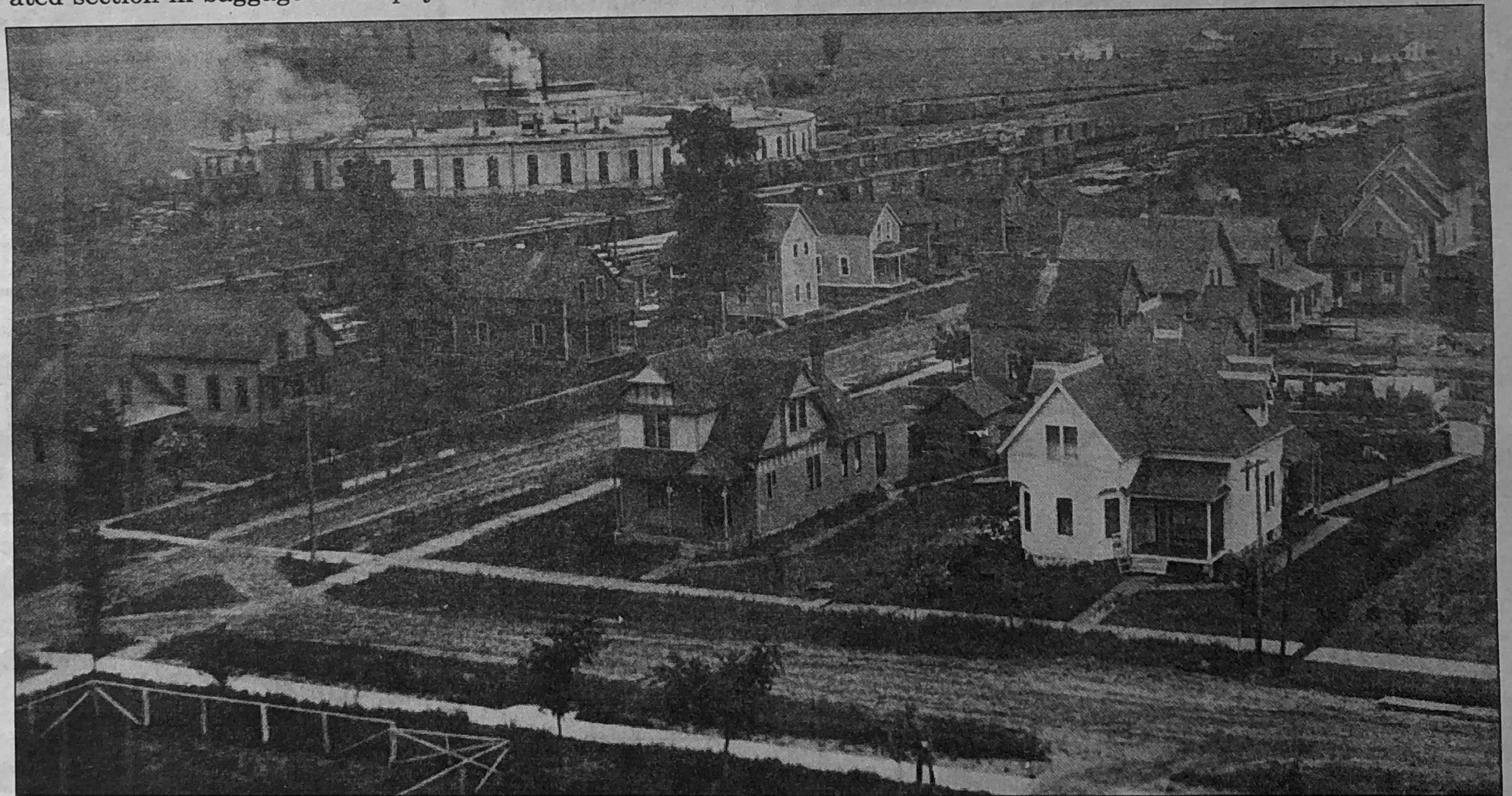
The roundhouse north of the courthouse was a landmark long after Antigo lost its prominence as headquarters to the Ashland division.
