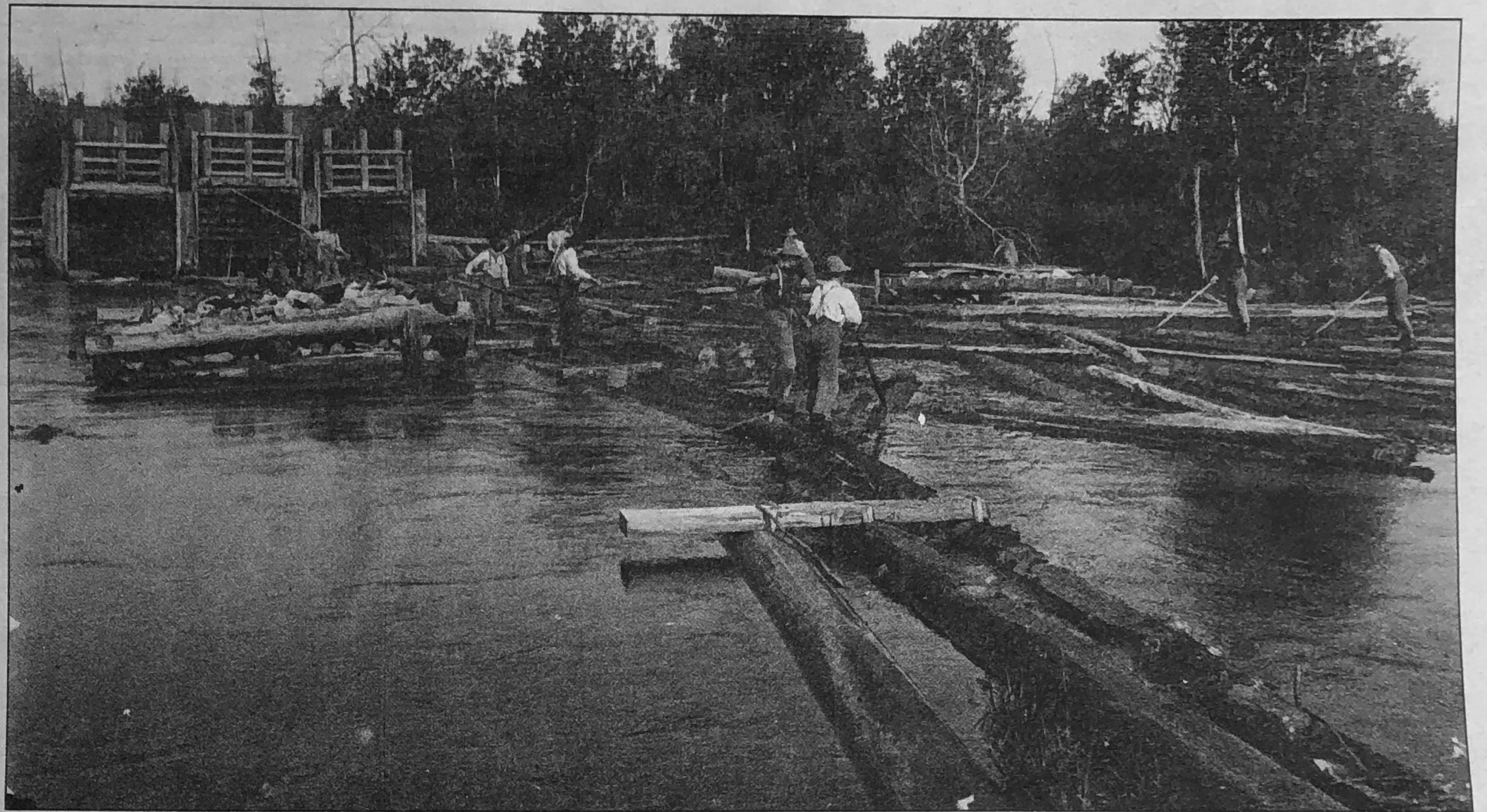
This dam on the Wolf is typical of many that controlled water flow during a drive.
