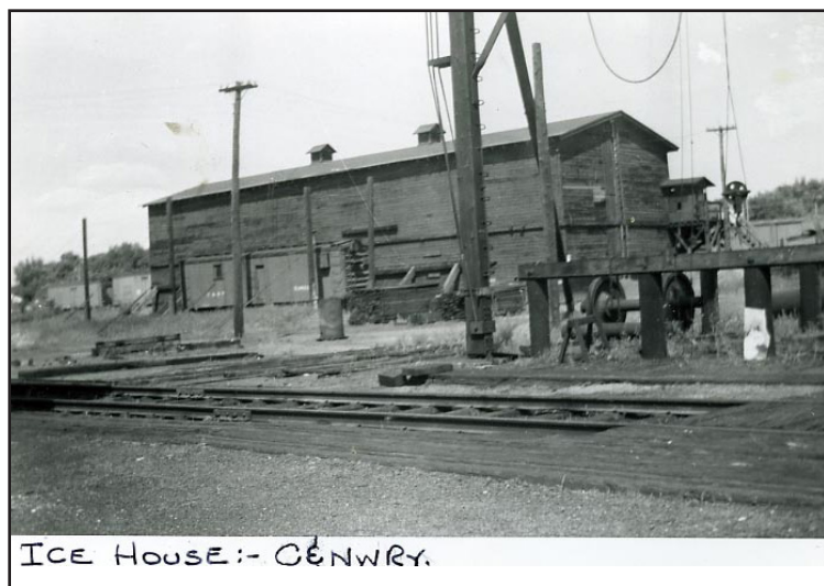
The ice house was adjacent to the tracks in the railyard. Cars would pull up beside it to be loaded with ice.
