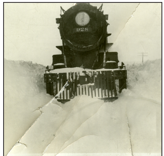
Engine 928 out of Antigo clearing the tracks after a snowfall
