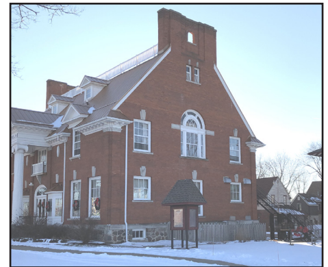
The north side of the museum will be undergoing a major transformation with the addition of a tower housing an elevator, restrooms, and an information lobby.
