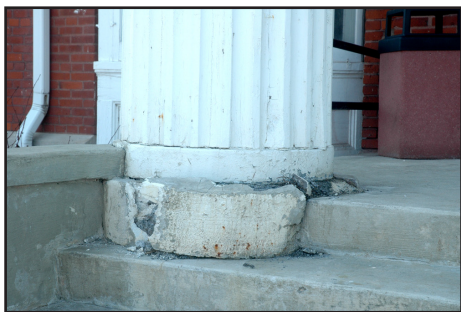
The front facade of the museum looks majestic but a closer inspection reveals badly needed repairs to the columns and stairs.
