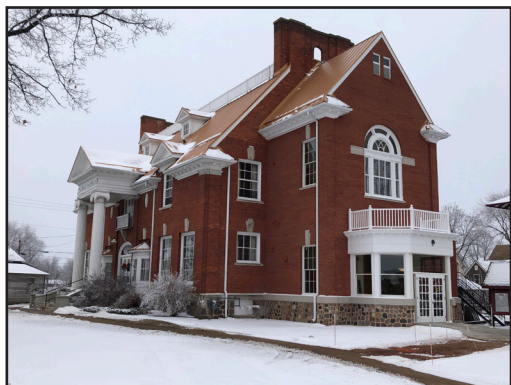
Nearing completion: the museum and its addition
